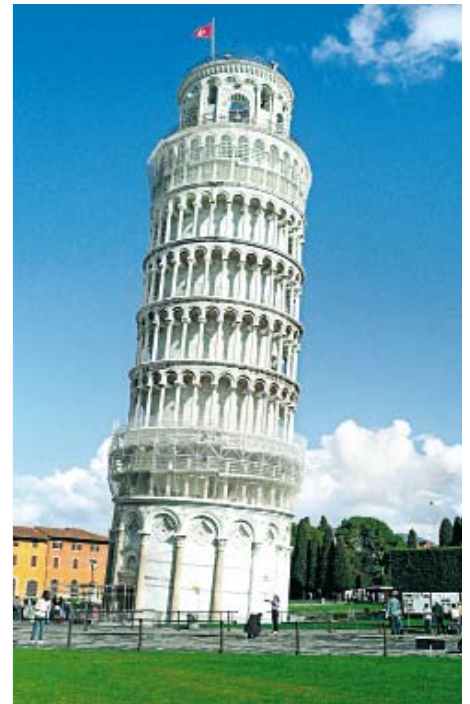
Leaning Tower of Pisa
